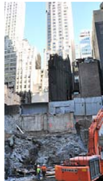
Close-in urban blasting in New York.
