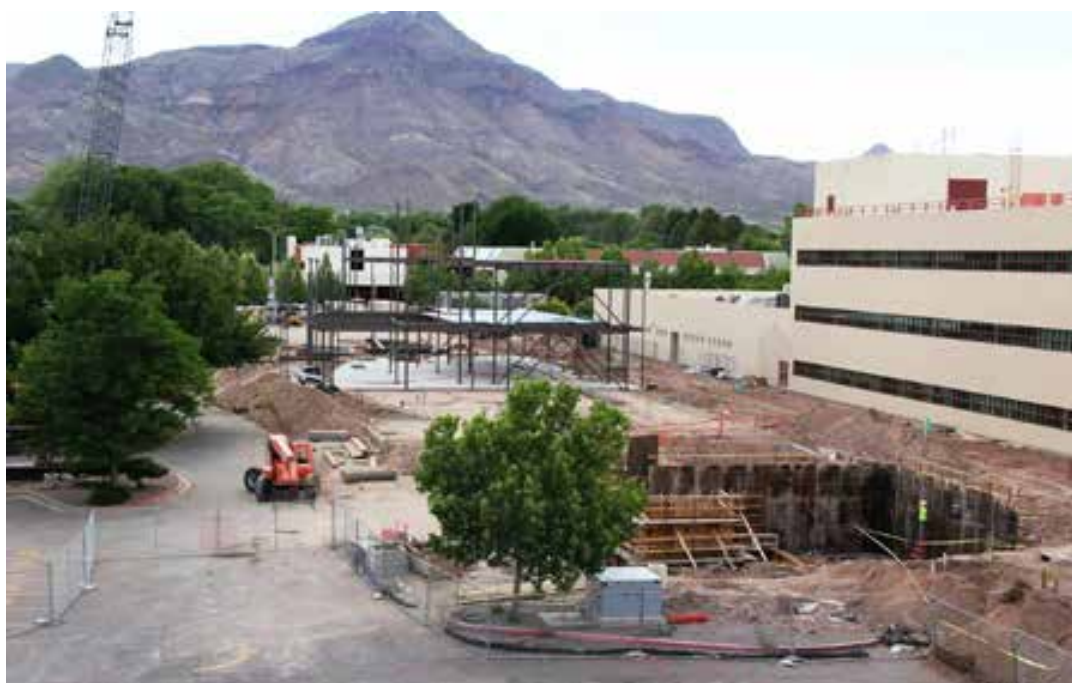
Construction site of the new Chemistry building
