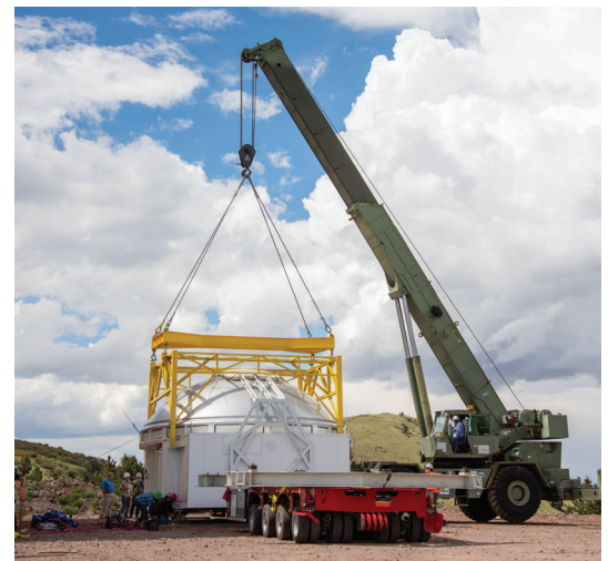
First telescope and enclosure being moved onto transport via crane to be located on the pad on the MROI array. Photo credit: Colleen Gino
